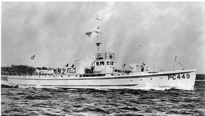
down 10 July 1939 as **PC-449** by the Luders Marine Construction Co., Stamford, CT; she was launched, 14 May 1940, and commissioned **USS SC-449**. This vessel was one of three Submarine Chasers built in a design competition. Although she possessed 50% more stability than the other prototypes, the contract would eventually be awarded to another firm, thus making her a one-of-a-kind.
